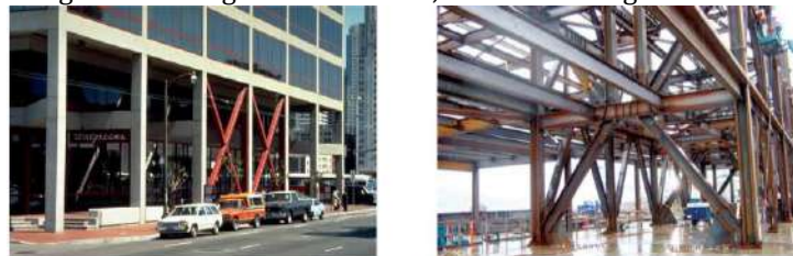
Fig 7. Steel bracing types include (a) eccentric bracings,
